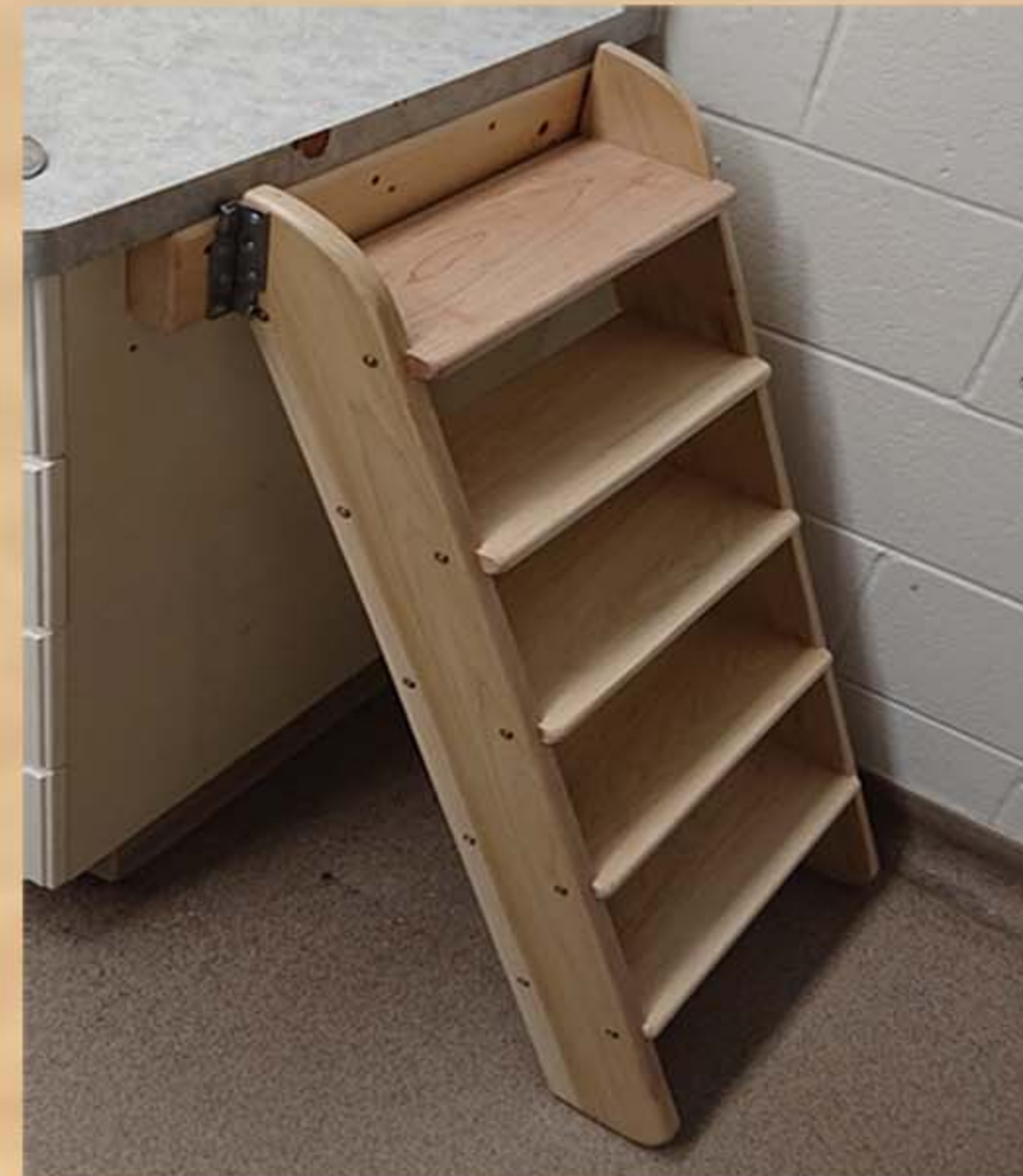
Steps to allow children to climb up to counter for diaper changes. Steps are removable.
